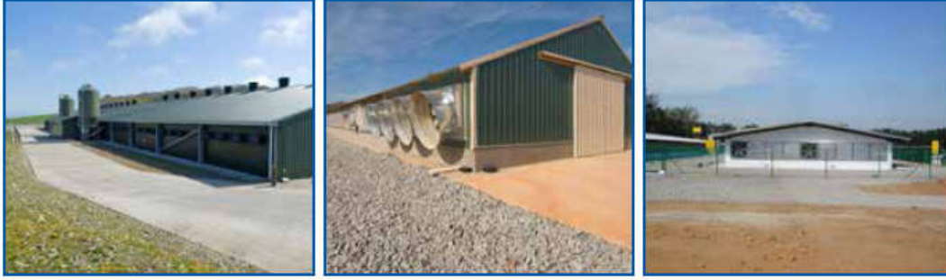
شكل (38) Houses with a low biosecurity risk showing concrete areas and no vegetation around the immediate perimeter of the house
