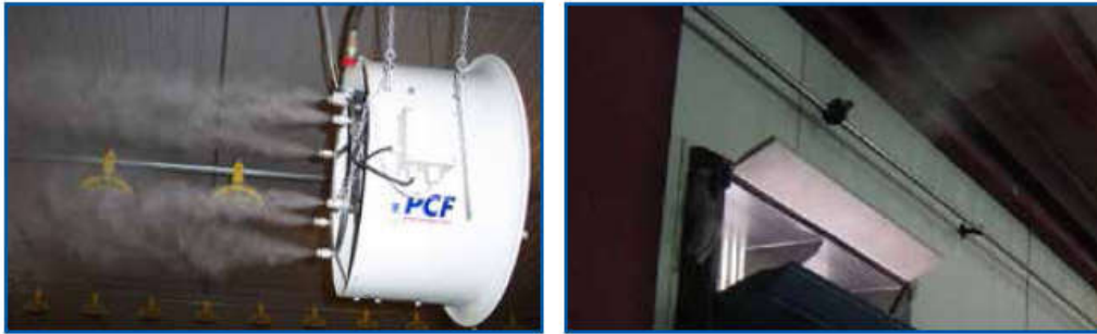
شكل (46) Use of a mister to increase RH during brooding
