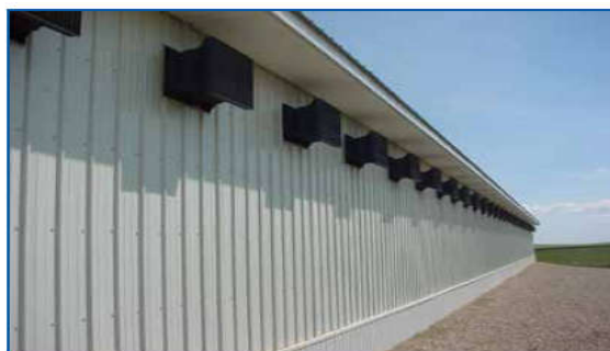
شكل (173) Example of a light baffle fitted to a cross ventilation inlet
