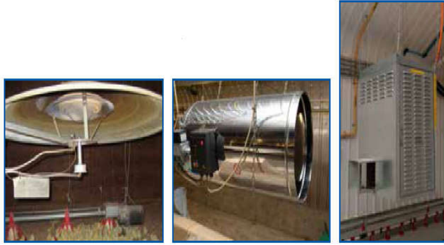
شكل (152) Example of different house heating systems (from left to right, canopy brooder, whole-house heating, and space heater)
