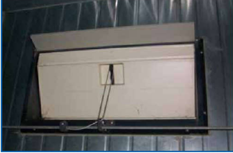
شكل (٣٩) Example of a good-quality air inlet
